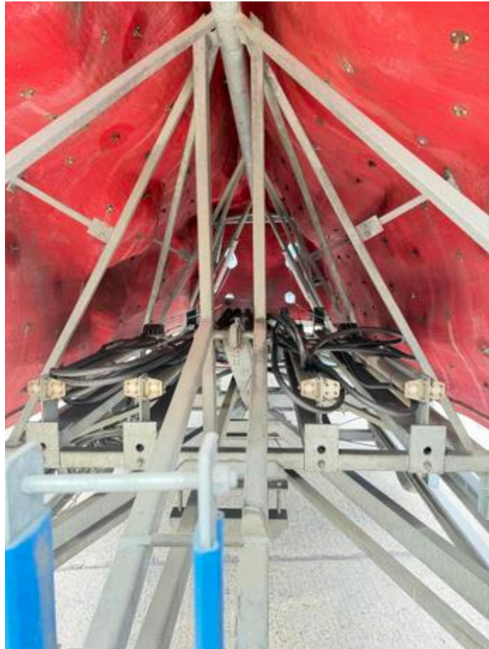
Photo of substructure if accessible or surrounding areas
